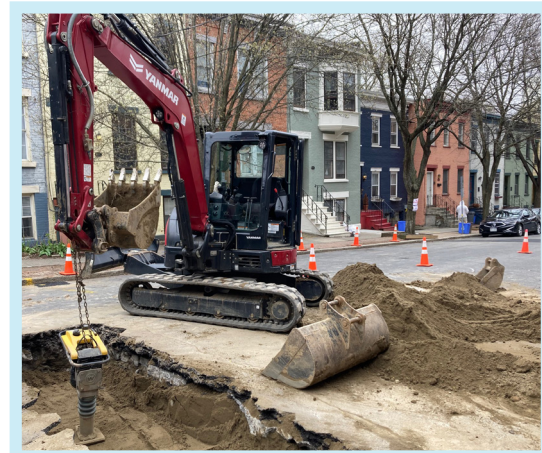
Photo 4: Lead pipe replacement in Albany.
