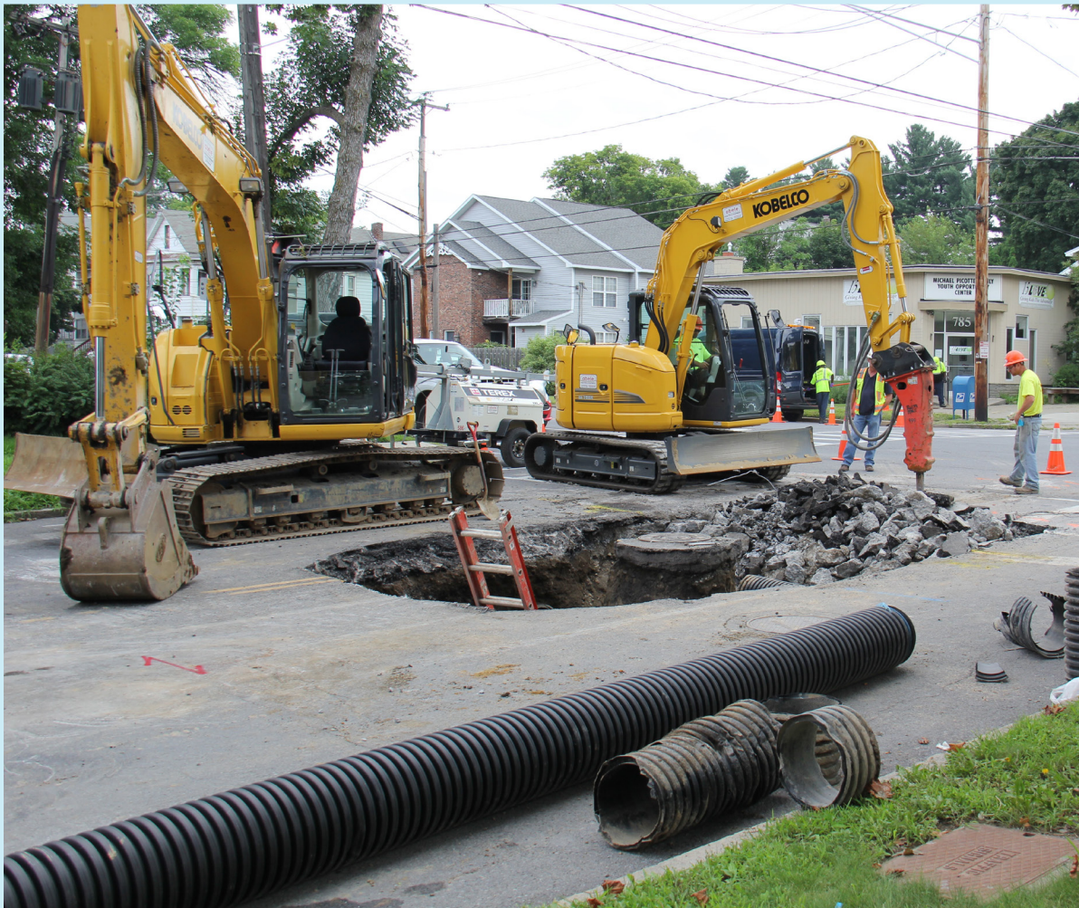
Photo 5: Water infrastructure upgradet in Albany.
